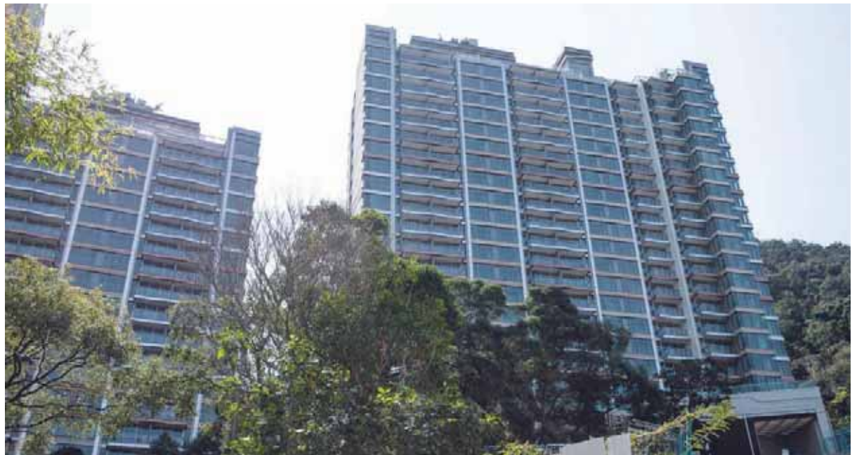
A man walks past a construction site on a road in front of residential buildings at 21 Borrett Road (top) in Hong Kong, where a five-bedroom, 3,378 square-foot penthouse flat has sold for $59.3 million. — AFP
