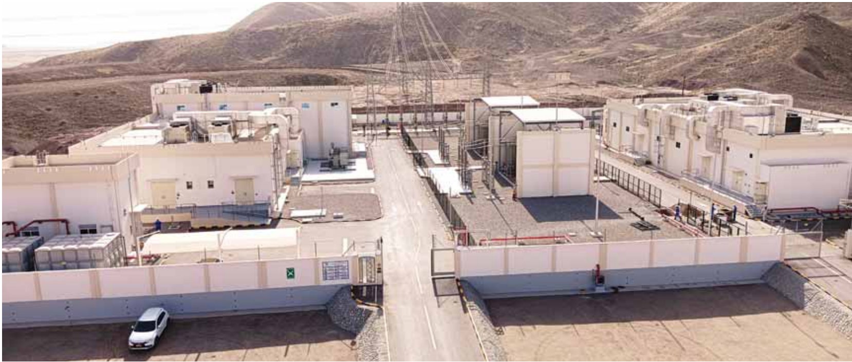
Oman Electricity Transmission Company has recently completed all construction and energisation work for the 132/33 kV Al Jawabi Grid Station.
