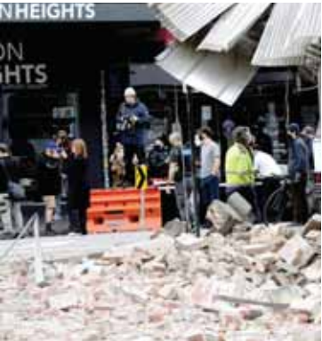
People gather near a damaged building in Melbourne after a 5.8-magnitude earthquake. — AFP
