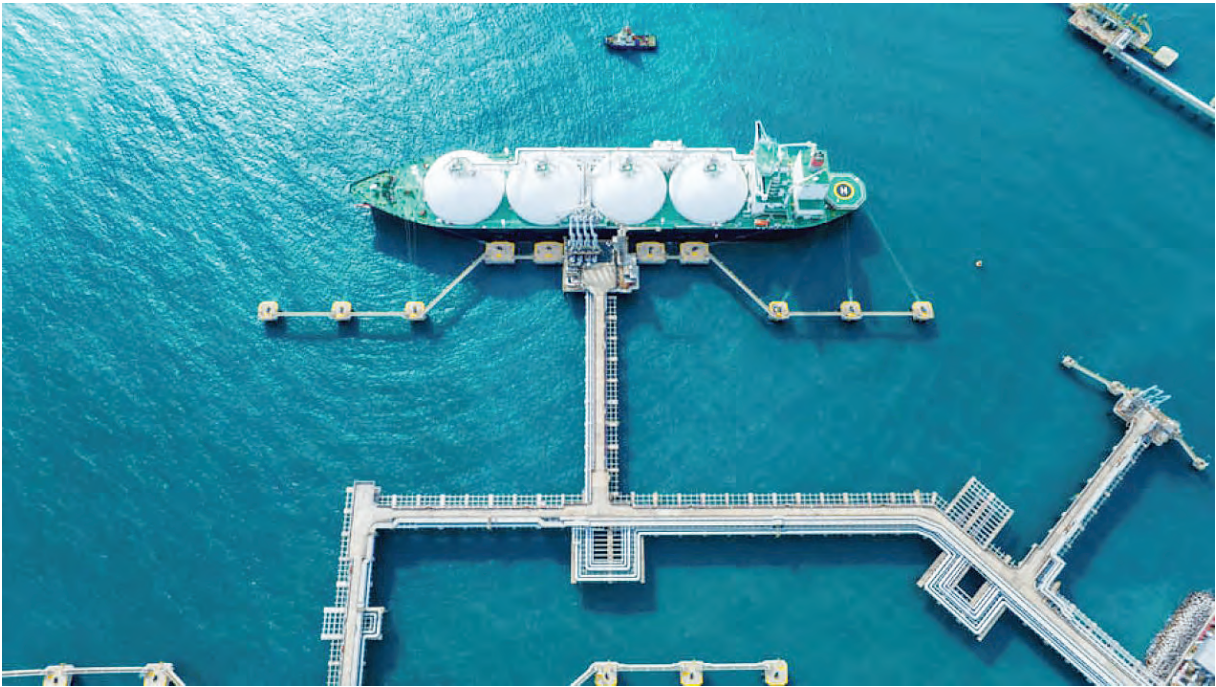
(Picture for illustration only) Amigo LNG is a 7.8 mtpa capacity liquefaction plant and export terminal located on Mexico's Pacific coast
