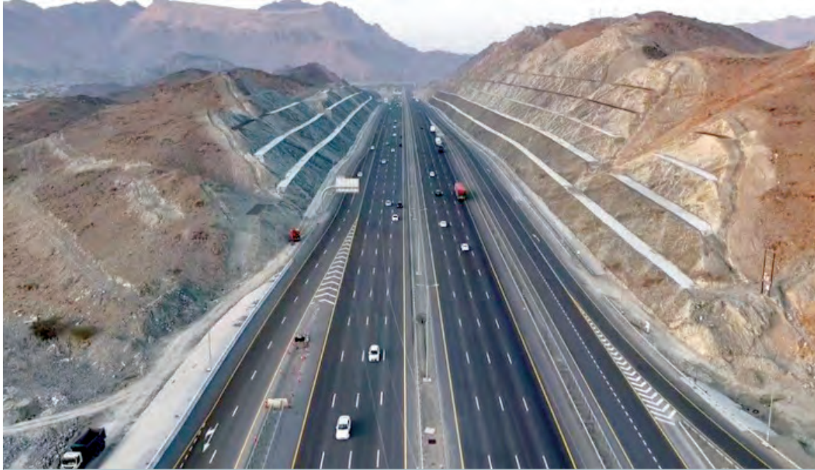
The Tender Board has awarded the contracts for the third, fourth and fifth parts of the Adam-Thamrait Road, along with the Jabal Shams Road, at a combined value of RO 278.452 million.
