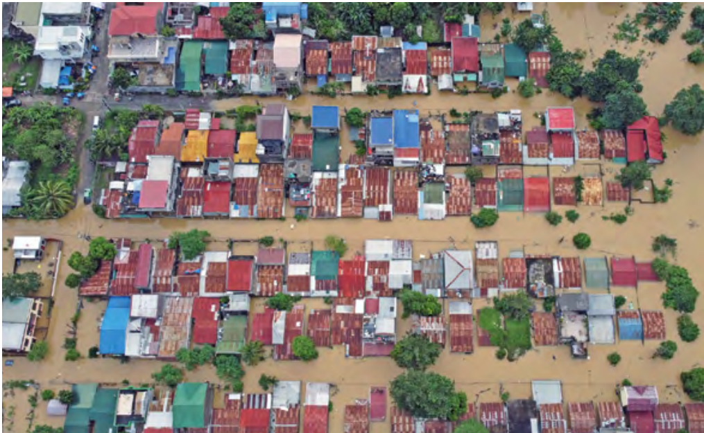
An aerial view shows flood-inundated houses at Capitol Hills in Alibagu, Ilagan city, Isabela province on Monday, after Tropical Storm Nalgae hit the region (AFP)
