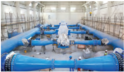
Al Dakhiliyah is witnessing the implementation of public service projects in the electricity, water and sanitation sectors. — ONA
