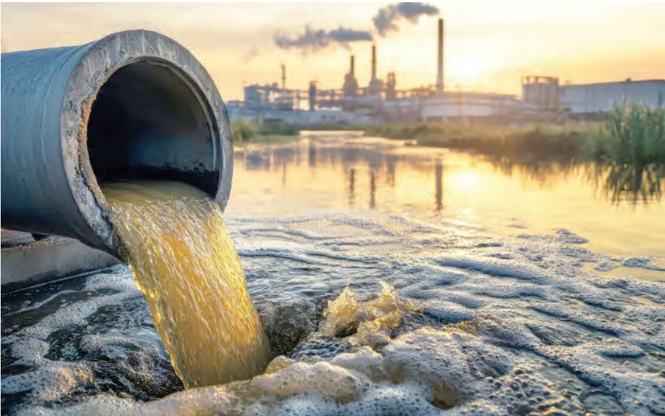
The study focuses on developing sustainable and effective methods for removing phenol, a hazardous pollutant commonly found in industrial wastewater.
