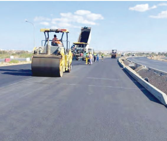
All works on the first section of the project have been completed. — ONA
