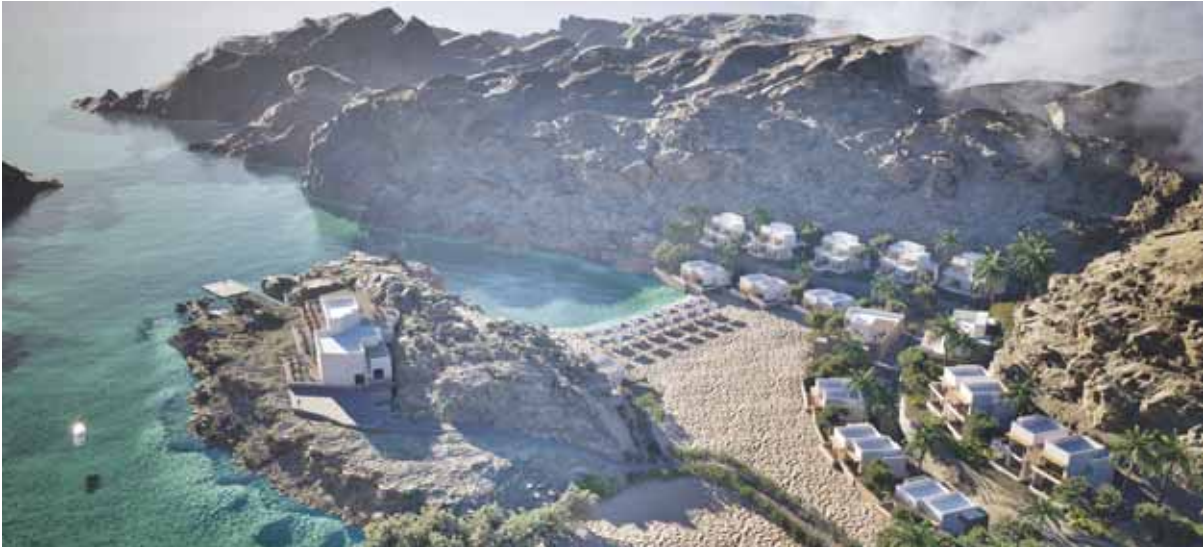
The RO 36 million project is located on the outskirts of Muscat.
