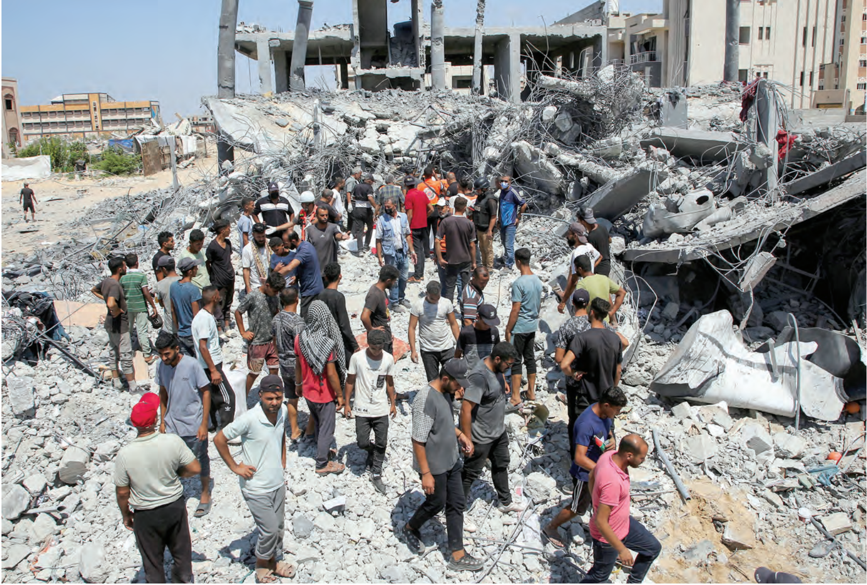
Palestinians inspect damage in Hamad City, following an Israeli raid, in Khan Yunis. — Reuters
