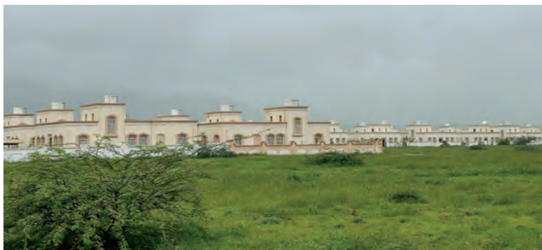
The Sahil Hamran housing project in Dhofar awaiting completion 18 years on.
