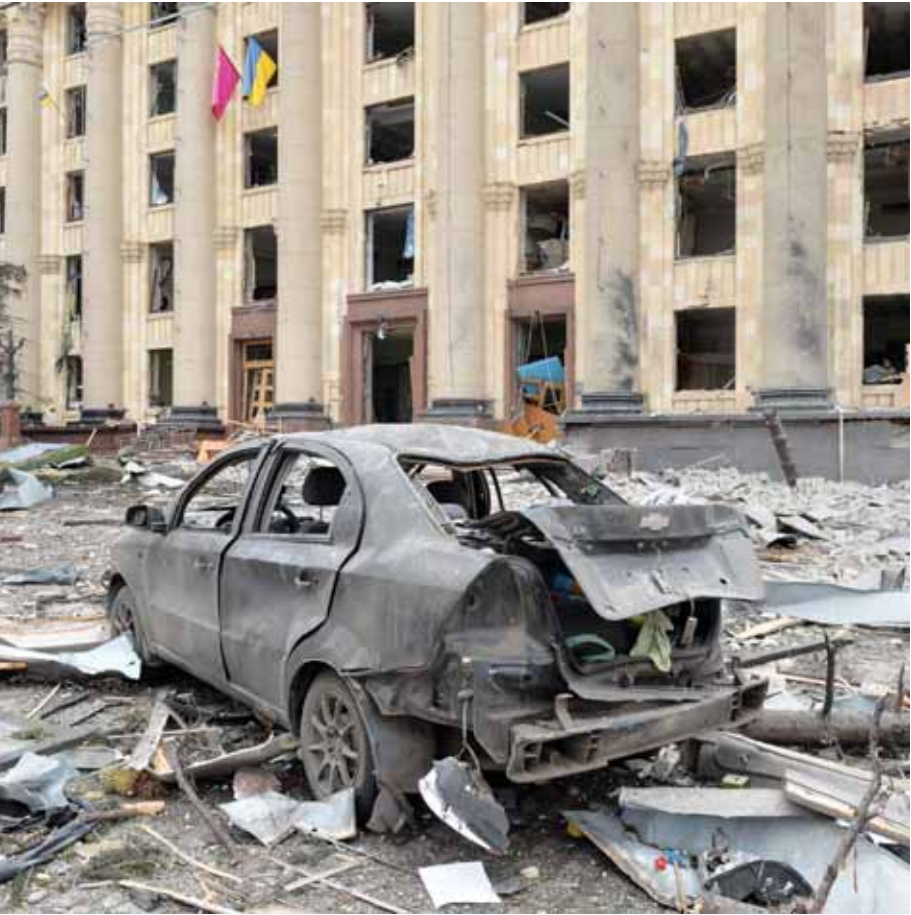
The damaged local city hall of Kharkiv destroyed as a result of Russian troop shelling. — AFP
