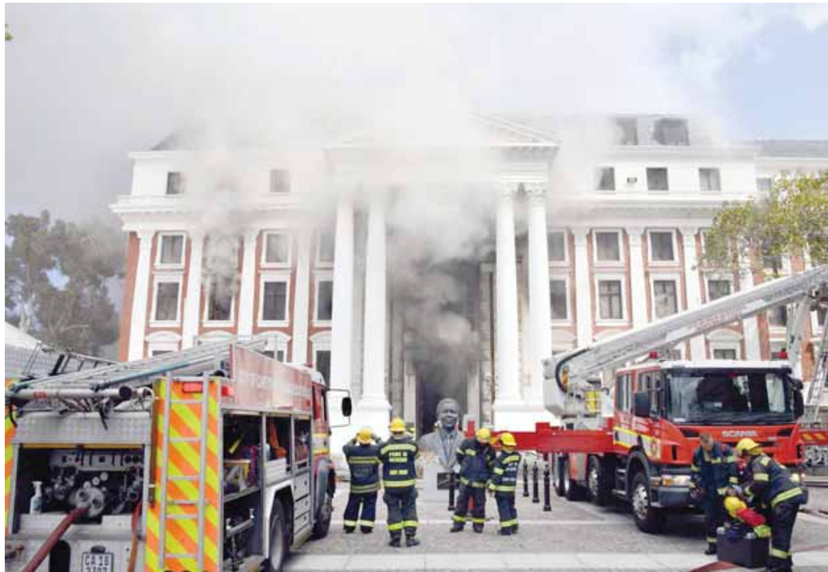
Firefighters battling the fire at the Parliament building in Cape Town. — Reuters
