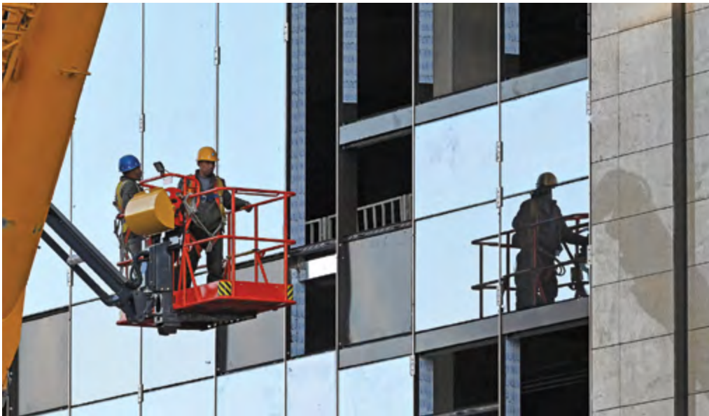
Workers prepare to install a window panel at a construction site in Beijing on Tuesday (AFP)
