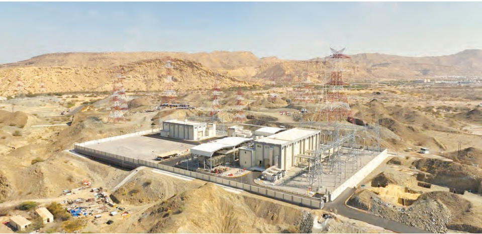
More than 60 per cent of the second phase of the Rabt project has been completed.
