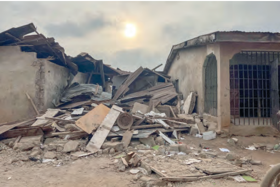
A general view of destroyed structures in Offa caused by debris from expended munitions that fell from US strikes on unspecified IS fighters in Nigeria. — AFP
