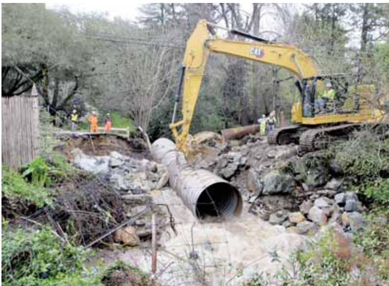
Workers install a new culvert after the road was washed out in an atmospheric river storm system in Soquel, California. — Reuters
