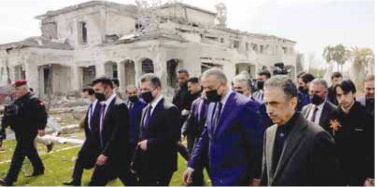
Iraqi Prime Minister Mustafa Al Kadhimi inspects a damaged building in Erbil. — Reuters
