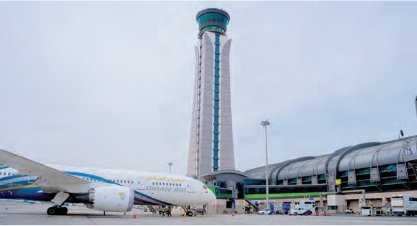
Operational teams at Muscat International Airport are working round the clock to ensure the smooth flow of passengers.
