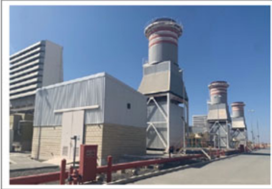
View of Three Gas Turbines
