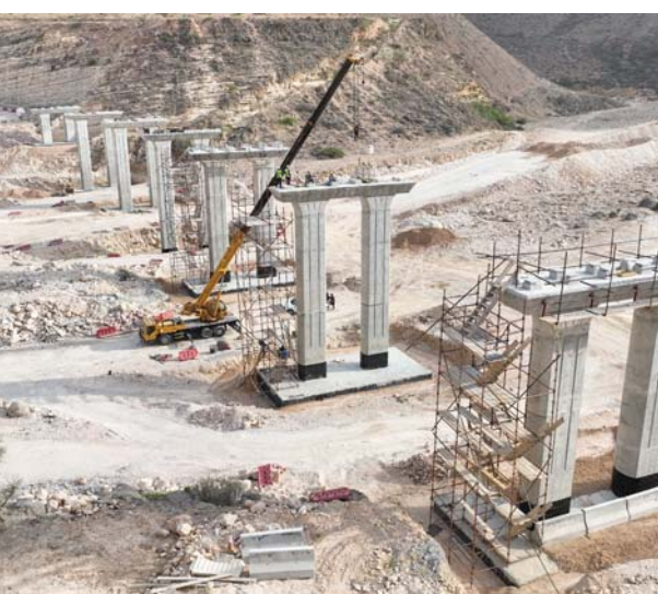
The Directorate-General of Roads and Land Transport has expedited road rehabilitation works at various locations within Dhofar Governorate including the annual maintenance project for the paved road network for a five year period at a cost of RO 3 million, the official said noting that
