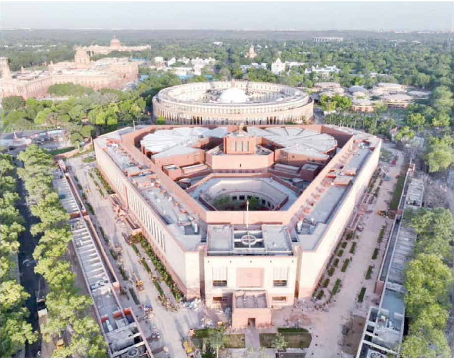
View of India’s new parliament building in New Delhi.
