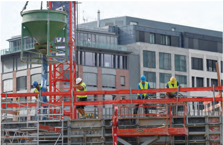
Construction sites are photographed in Frankfurt, Germany. — Reuters
