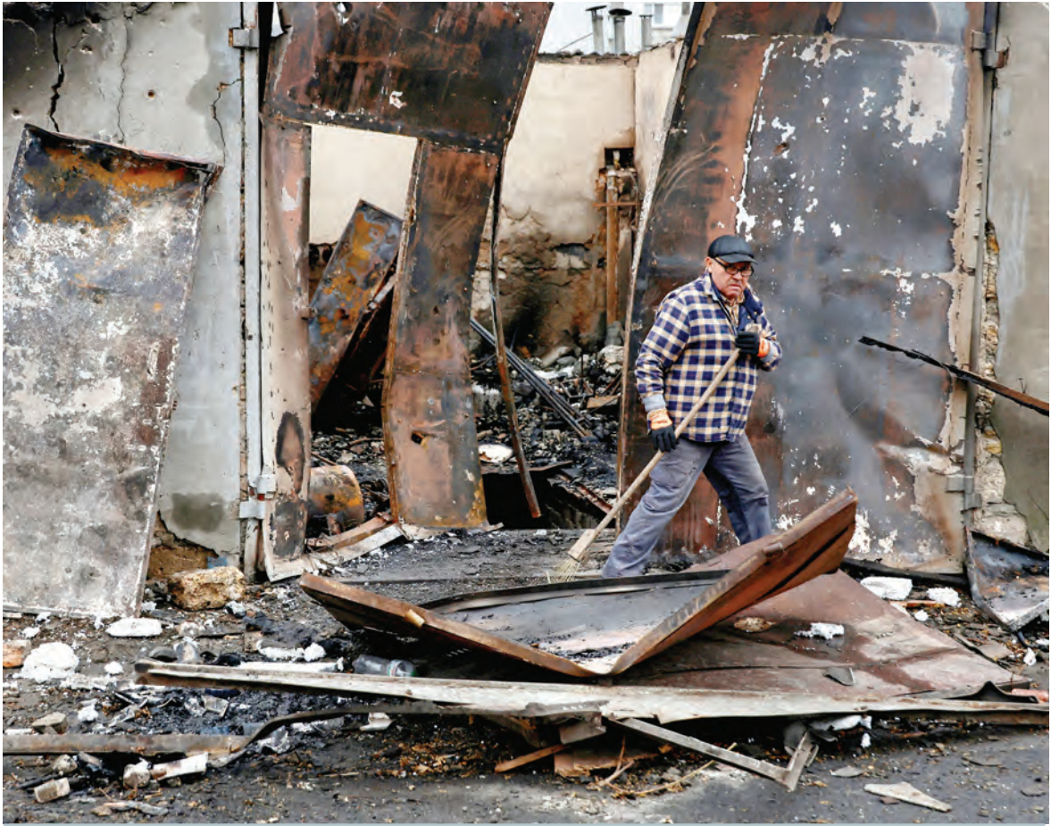
A resident removes debris from a garage heavily damaged by a Russian drone strike, in Odesa. — Reuters
