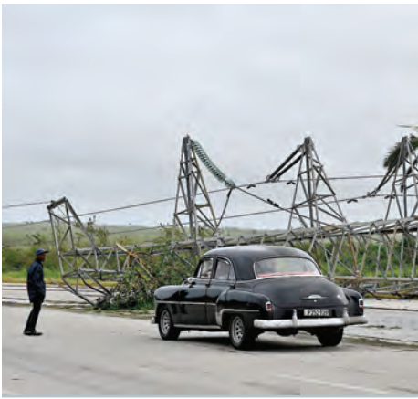
A car drives past a high tension electric tower knocked down during the passage of Hurricane Rafael on the road linking Artemisa with Havana. — AFP
