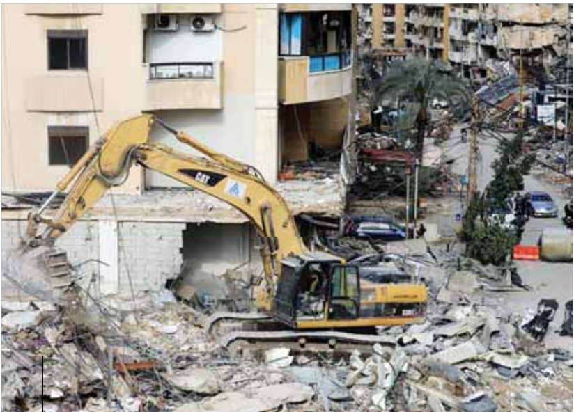
View of Lebanon after Israel-Lebanon ceasefire deal A man operates an excavator to clear the debris in the southern suburb of Beirut, Lebanon. According to the ceasefire deal, the Lebanese army will take control of southern border areas over the next 60 days, Israel will gradually withdraw, and civilians will return home. Xinhua
