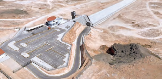
The Wadi Al Khoudh project forms part of the wider Climate-Resilient Flood Protection Dams Project, backed by IsDB financing (Picture for illustration).
