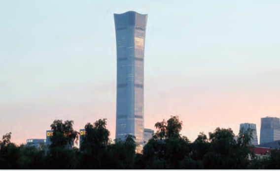
The CITIC Tower, where damage is visible on a high floor of the exterior, in Beijing. — Reuters
