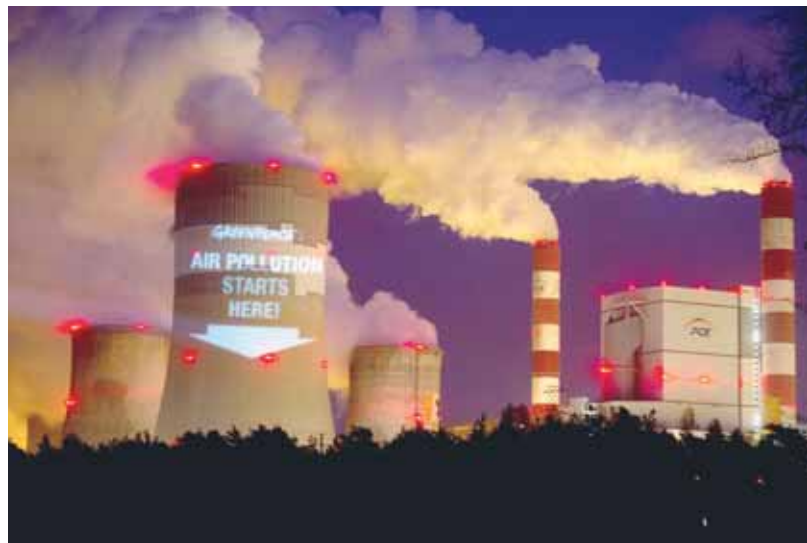
Greenpeace activists project a slogan onto the cooling tower of the brown coal fired Belchatow power plant, in Belchatow, Poland. — Reuters file photo
