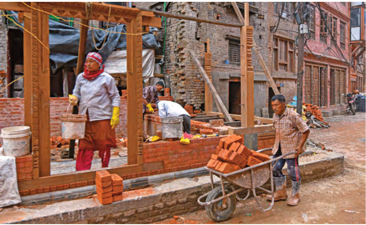
Labourers work to reconstruct a temple in Bhaktapur on the outskirts of Kathmandu
