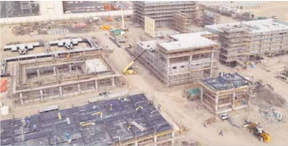
All major buildings have been completed and are ready to receive the necessary equipment, with installations scheduled to begin in mid-September.
