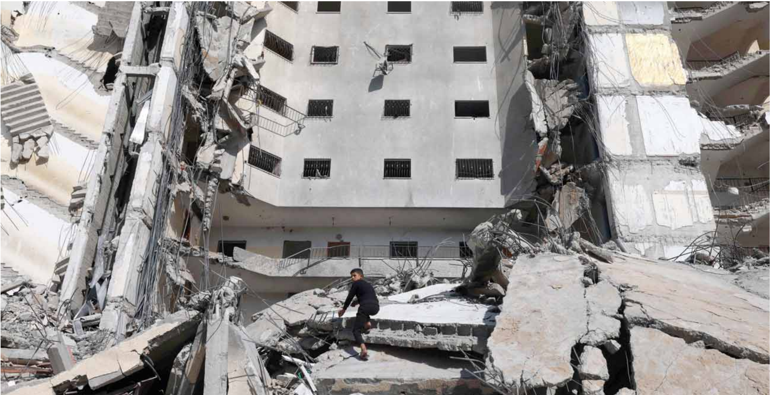
A Palestinian boy inspects the damage to a building hit in an Israeli strike in Rafah, in the southern Gaza Strip. – AFP
