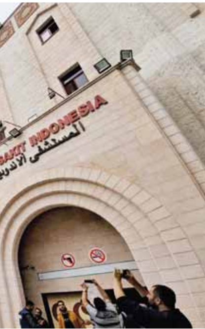
of fuel and electricity, in the northern Gaza
