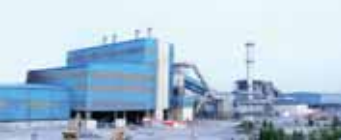
View of Oman's first ferrochrome smelter, which was launched at SOHAR Freezone in 2013.
