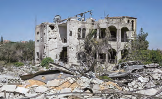
A photograph shows the damage in Zawtar Al Gharbiya, Lebanon. — AFP
