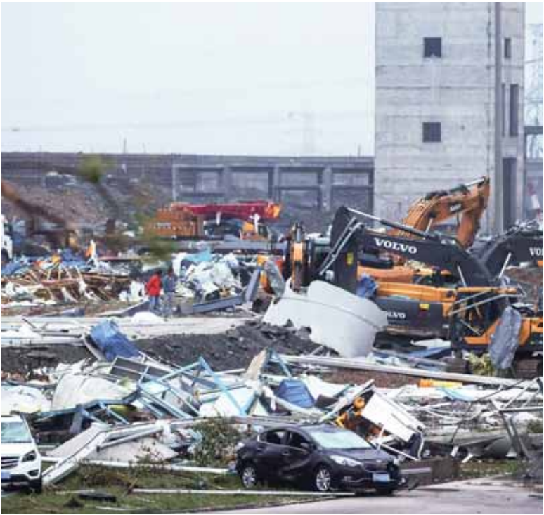
Damaged vehicles and debris at a construction site after a tornado hit an economic zone in Wuhan in China's central Hubei province. — AFP
