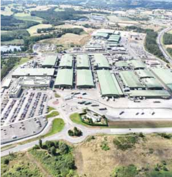
SNF's plant in Andrézieux, France.
