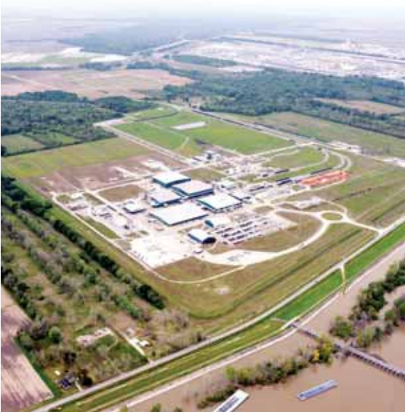
SNF's project facilities in Plaquemine LA, USA.
