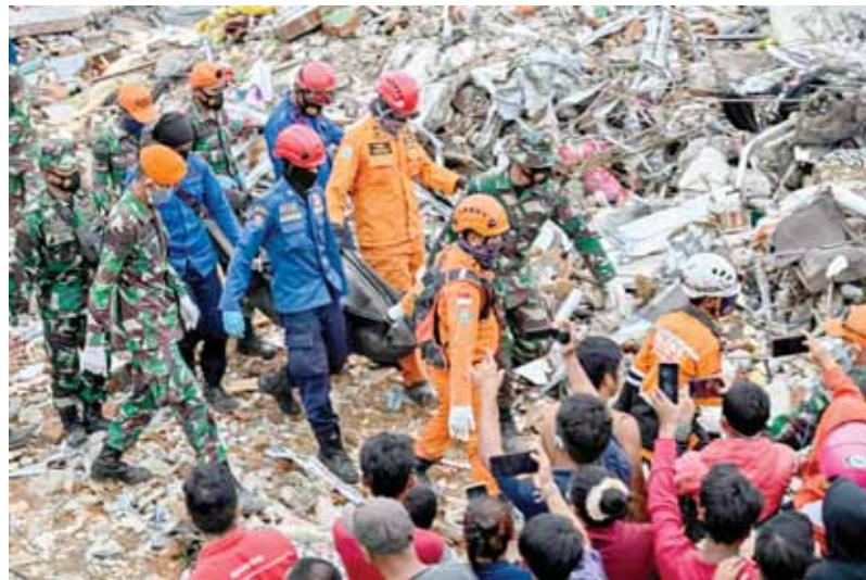
Rescuers move the body of a victim that was trapped in a collapsed building in Mamuju a day after a 6.2-magnitude earthquake rocked Indonesia's Sulawesi island. — AFP
