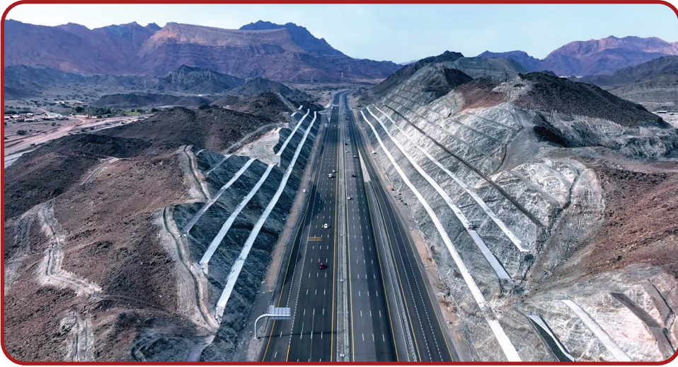
Oman's road network reflects the country's infrastructure development to the highest safety standards
