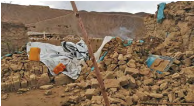
The earthquake caused massive damage to houses, says Badghis official
