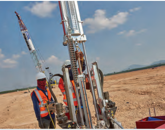
The fieldwork included deep and shallow borehole drilling, Cone Penetration Testing (CPT), and detailed assessments of pipeline routes and marine anchoring points. Image for illustration only.
