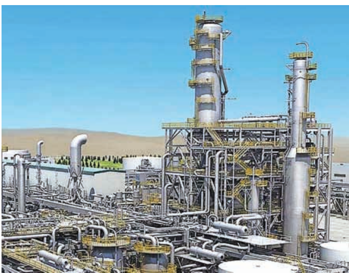
Strong growth is expected in number of ammonia plants in this decade
