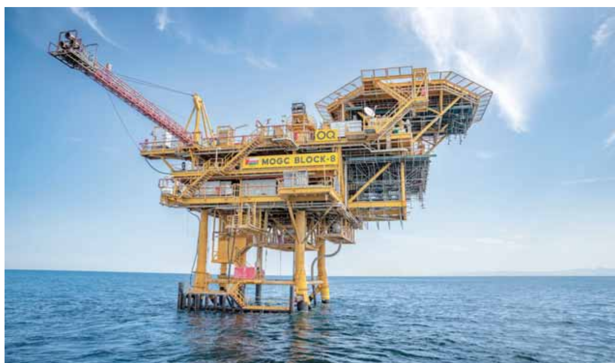
In the oil and gas sector, preventive measures protect facilities and workers from environmental accidents and leaks, covering onshore and offshore production plants, pipeline networks, and petroleum refineries.
