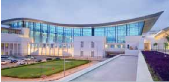
At Salalah International Airport, Acciona is targeting a 50% reduction in electricity consumption by replacing all lighting systems with energy efficient devices.
