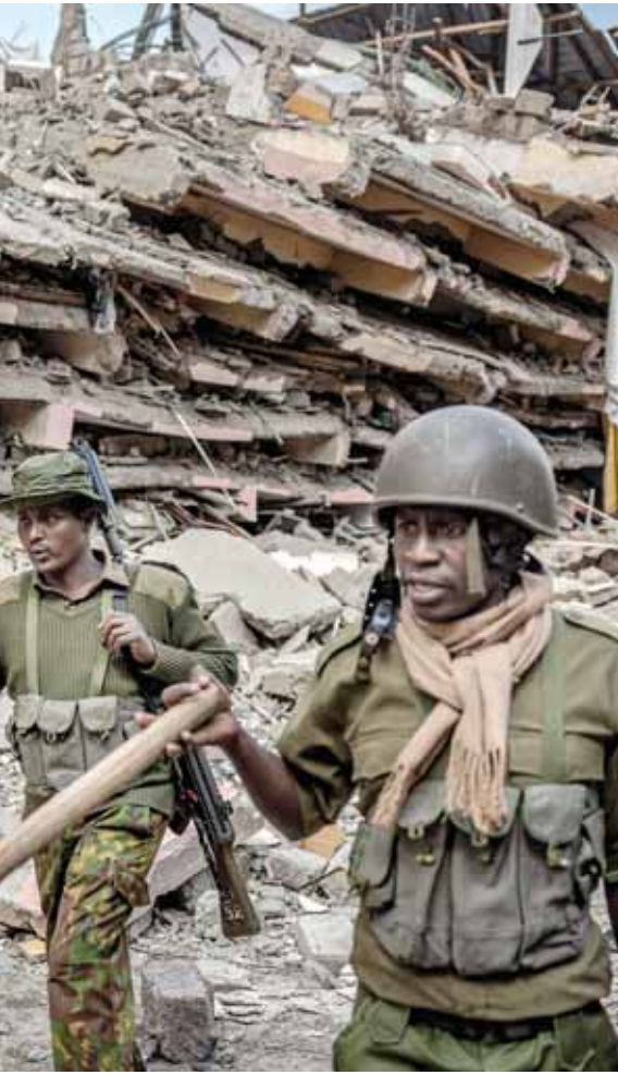
Kenya police officers give instructions to bystanders to evacuate the area next to a collapsed residential building at Kahawa West residential area in Nairobi. Response teams were responding to a building collapse in Nairobi. — AFP
