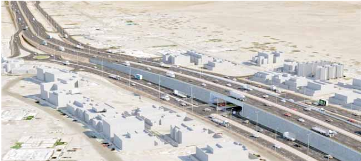
Muscat Municipality will embark on an expansion of Al Ansab-Al Jifnain road (phase 2) in the first quarter of 2023. The project aims at boosting the efficiency of the road by constructing three lanes in each direction from Falaj Al Sham in the Wilayat of Bausher to Al Al Jifnain in the Wilayat of Al Seeb as well as converting existing roundabouts into tunnels and flyovers.
