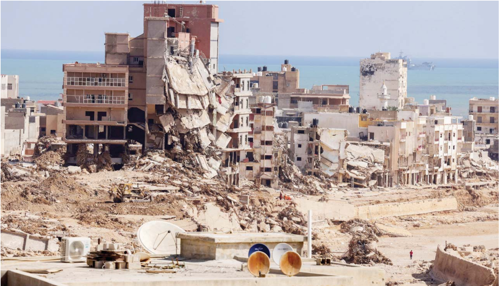
A view shows destroyed buildings in the aftermath of the deadly storm that hit Derna, Libya. — Reuters file photo
