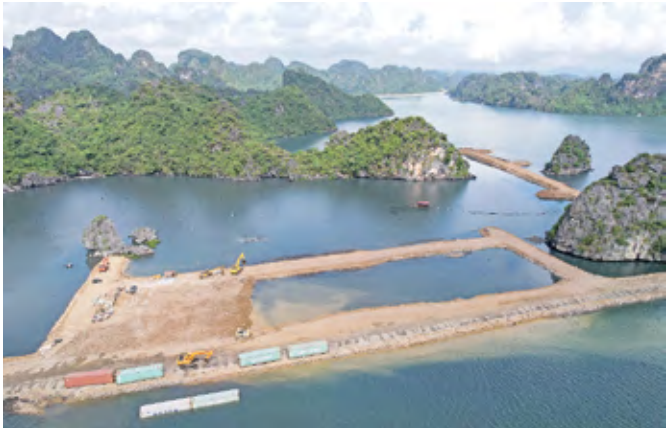
The construction site of a residential and hotel complex near Ha Long Bay in Vietnam's Quang Ninh province (AFP)
