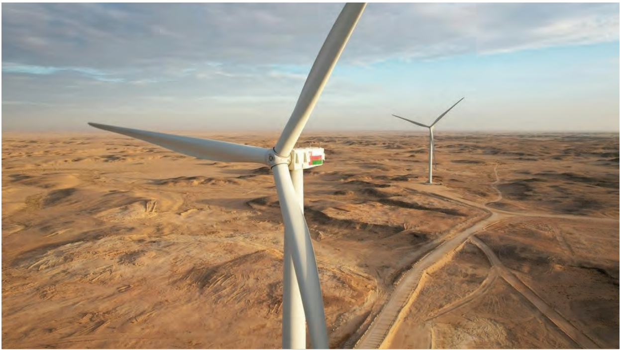
Omani multidisciplinary architectural and engineering consultancy Design Group Engineering Consultants (DGEC) oversaw the electrical design scope for the two wind energy packages.
