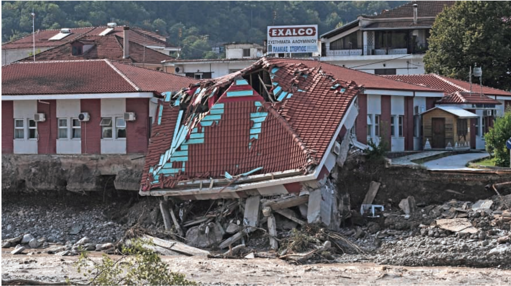
A heavily damaged health centre after the floods caused by the Mediterranean hurricane (medicane) Ianos hit the central Greek town of Mouzaki on Sunday (AFP)
