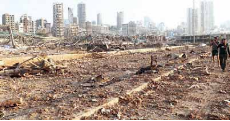
A view shows damages at the site of an explosion in Beirut. — Reuters File Photo
