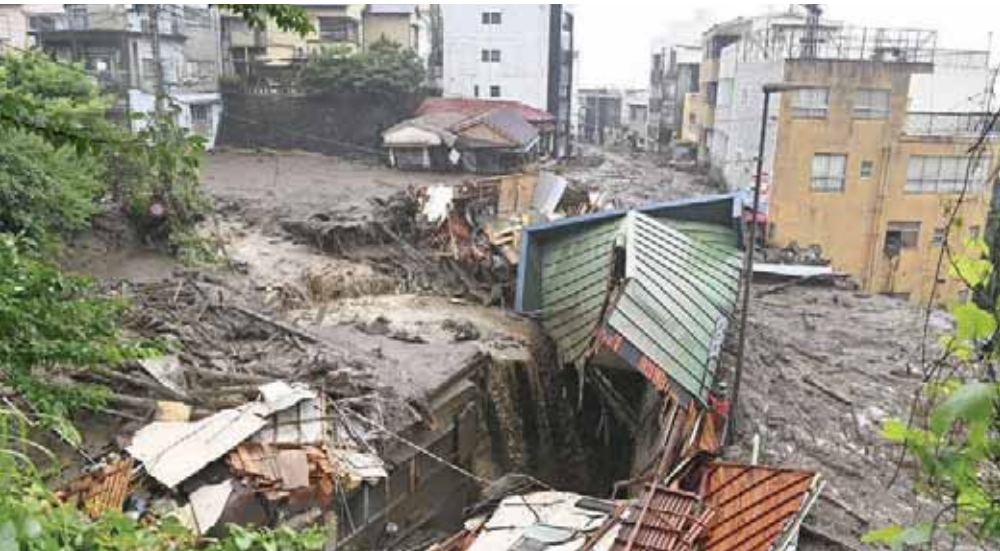
Houses damaged by a mudslide following heavy rain are seen at Izusan district in Atami. — Reuters
