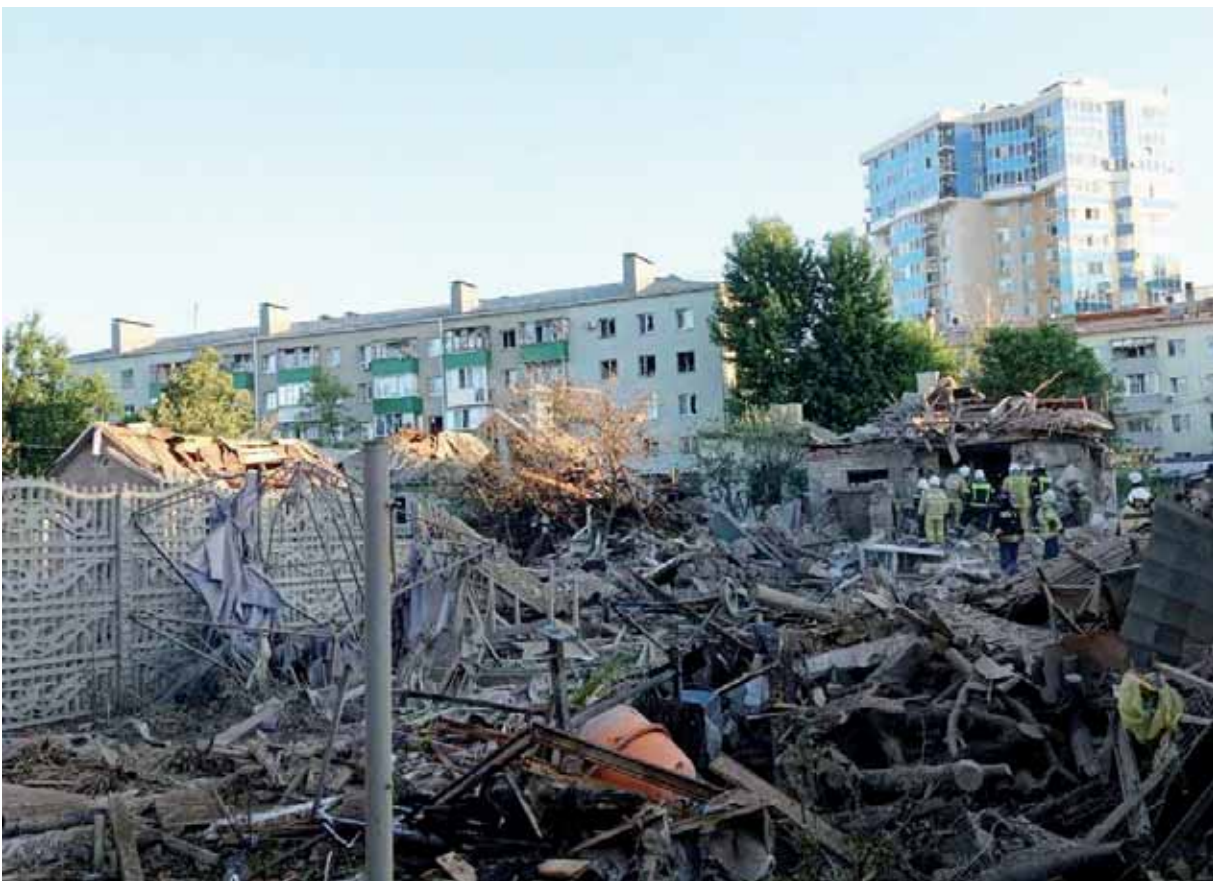
Rescue specialists work at the site of a destroyed residential building after the blasts in Belgorod, Russia. — Reuters
