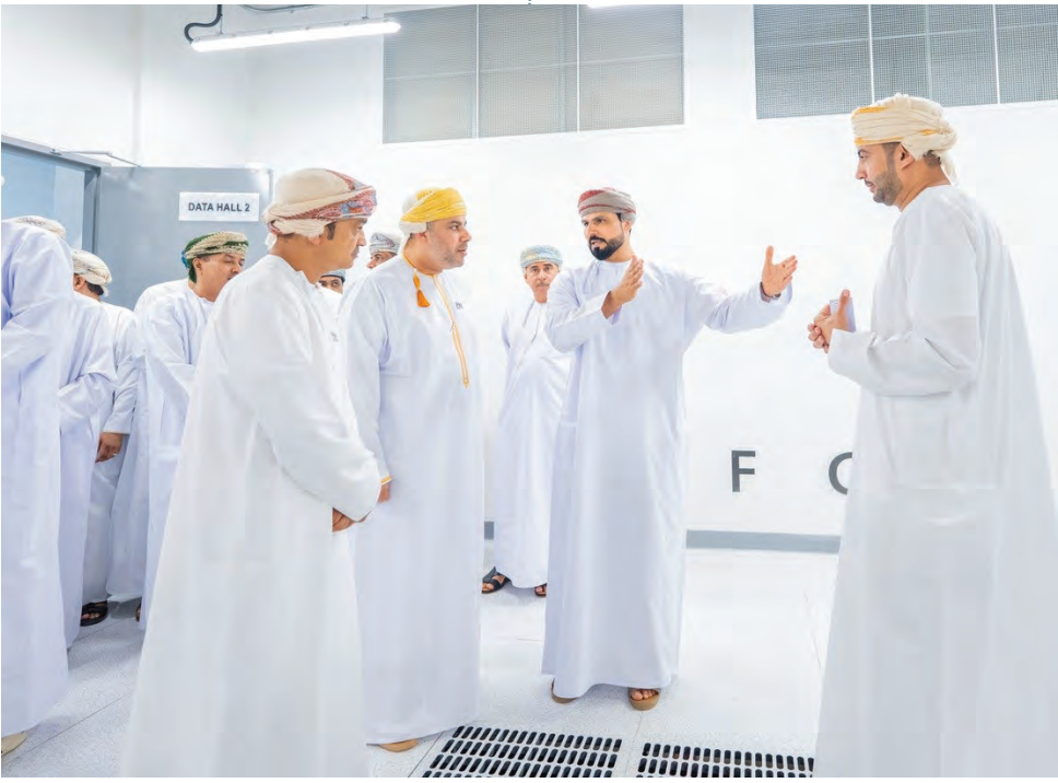
The new facility is the first of its kind in southern Oman to combine class 3 compliance data centre with a submarine cable landing station.
