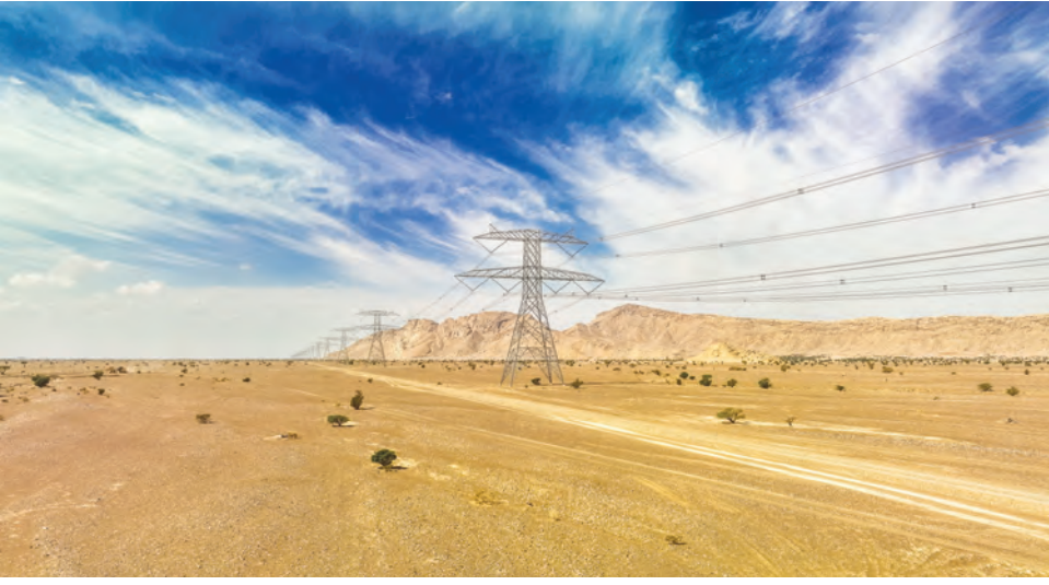
This achievement spans various work sites and projects across Oman.
