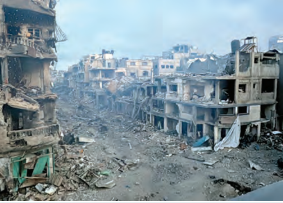
Palestinian houses stand badly damaged during the ongoing Israeli strikes in Beit Lahiya. — Reuters
