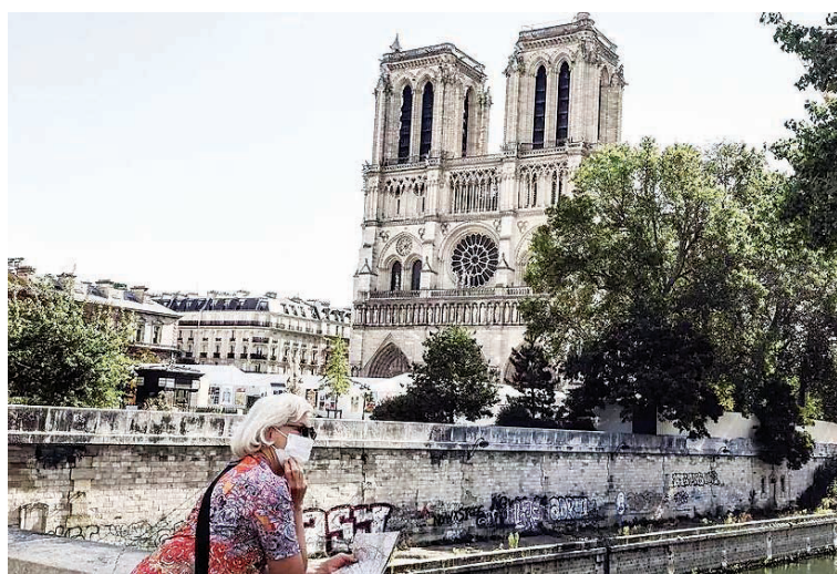
Notre-Dame restoration work has been plagued by delays. — AFP
