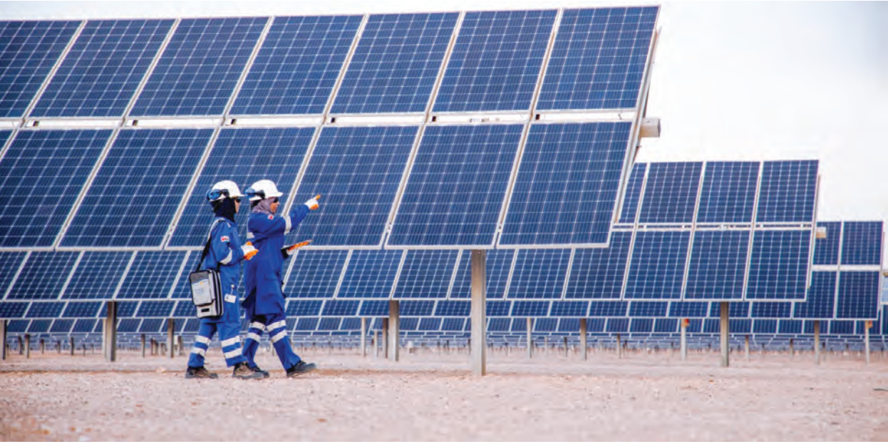
The solar IPPs are designated as Projects Number 11 and 12 under PWP’s renewable energy roadmap.
